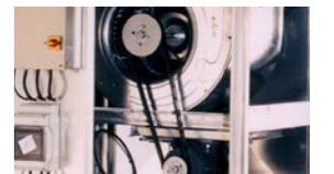
Centrifugal fans in RVH for high external pressure
